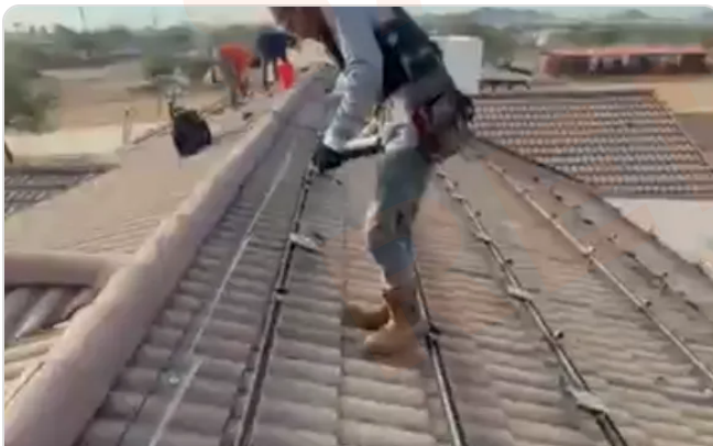
Racking, conductor routing and clamps inspected on the roof
