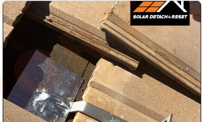
Representative mount: flashing and sealant intact
